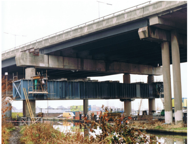
R53 – involving the installation of a 125te Plate Girder system
