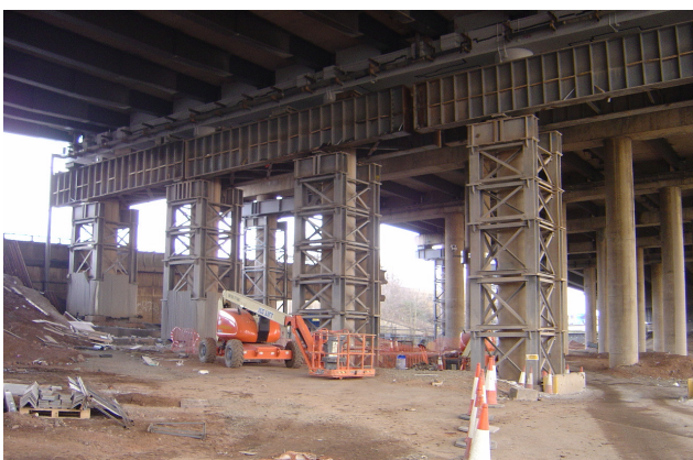
R121 – involving the installation of a 200te Plate Girder system
