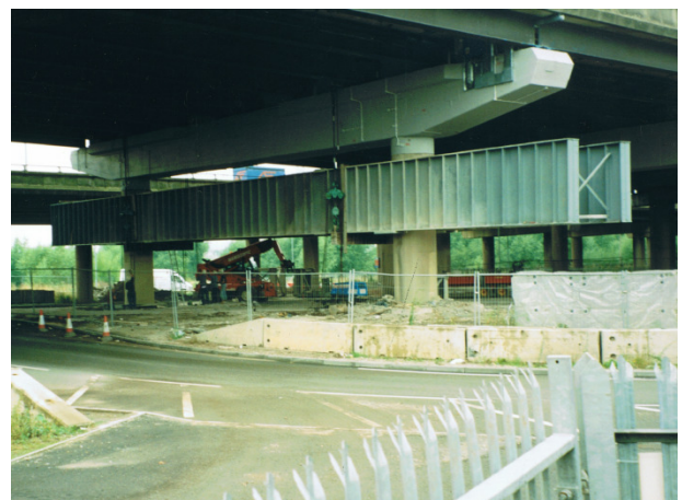
R97 – involving the installation of a 85te Plate Girder system
